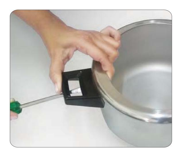
Unscrew existing handle. Screw on the replacement Subsidiary Body Handle. For best results, use a 6 mm tip screwdriver (not supplied in the Kit).
